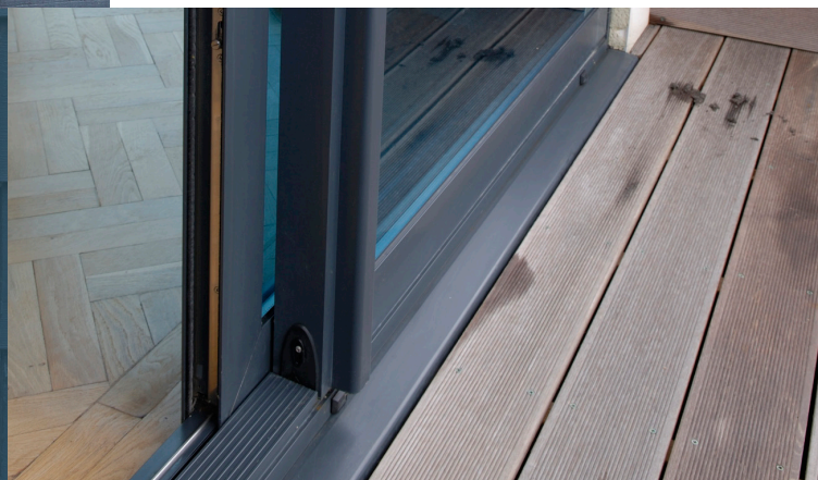
Twin Track Sliding Doors
